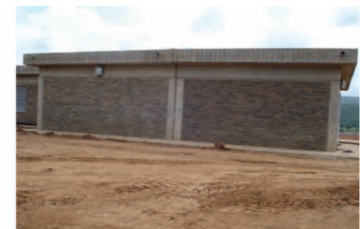
Zulu Crèche with VIP and Fencing
